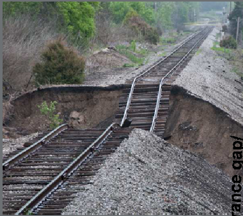
Railway embankment along Plymouth
